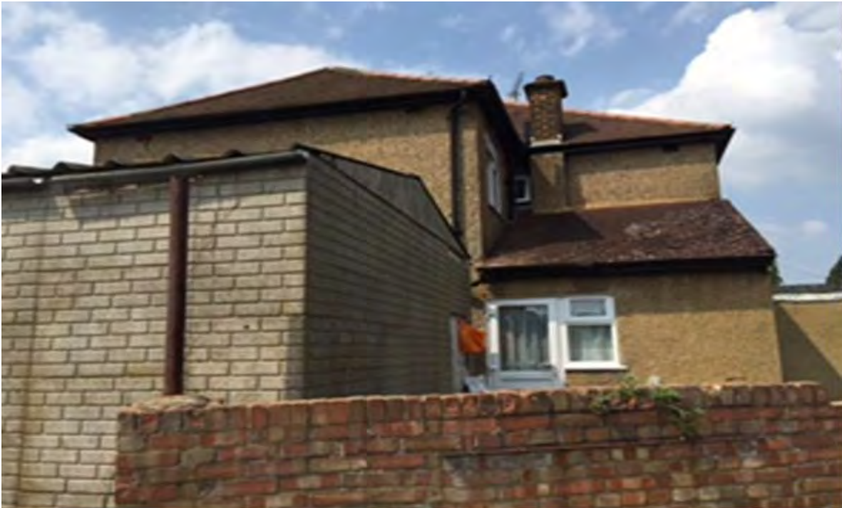
Side to rear elevations
